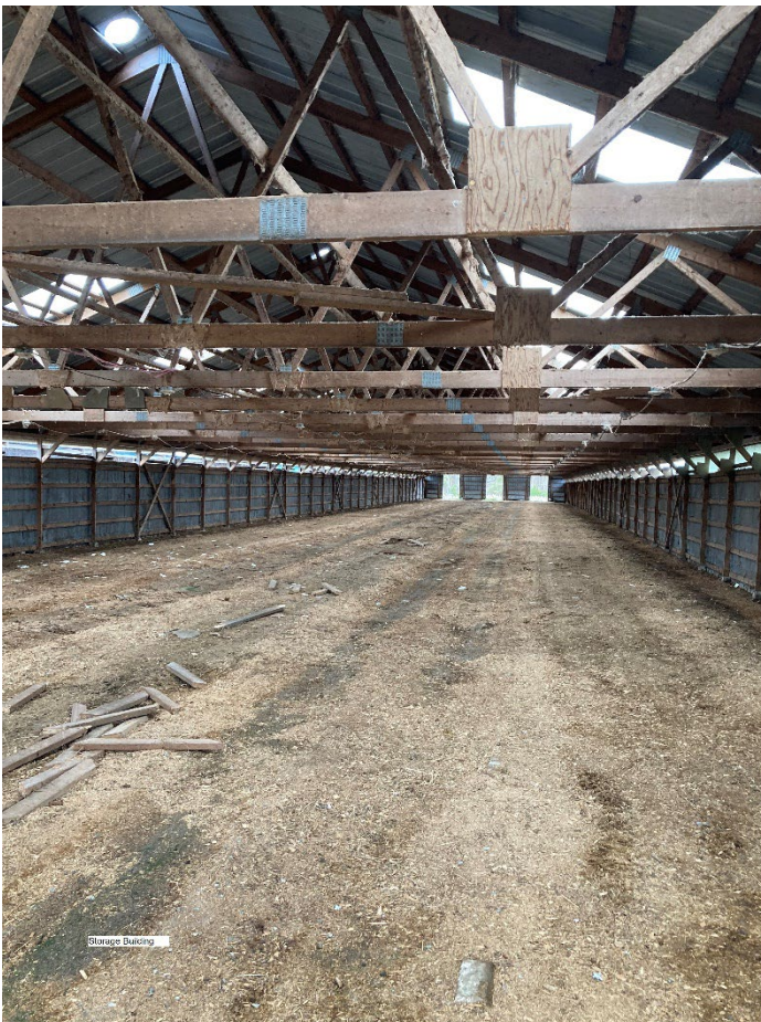
Interior of Warehouse/Storage Buildings
