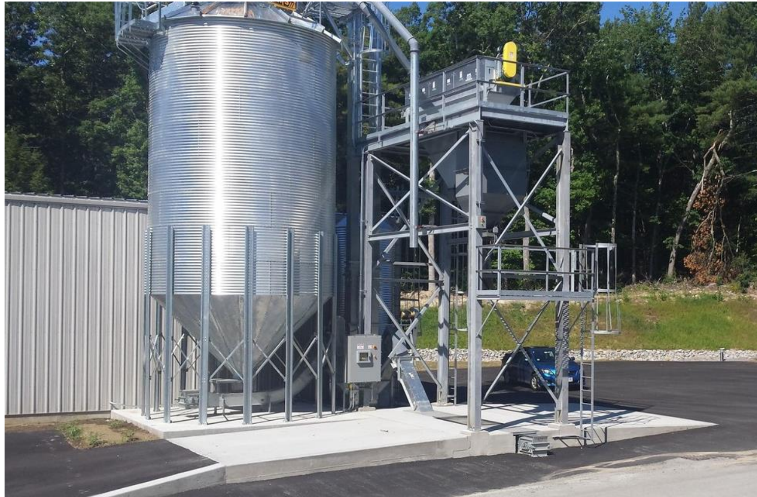
100 t pellet silo and filling facility in Massachusetts
